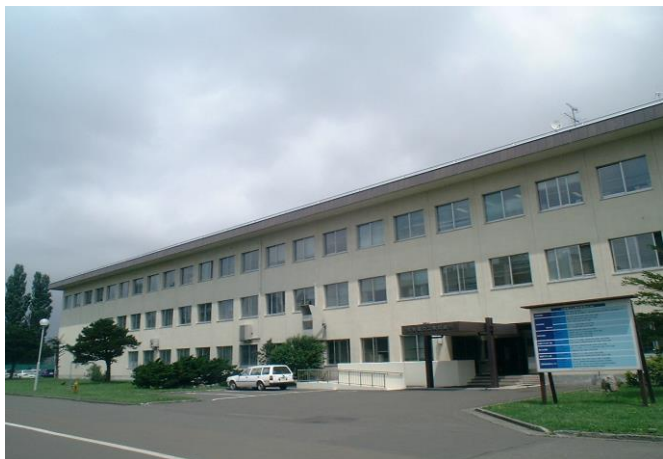
Appearance of Building
