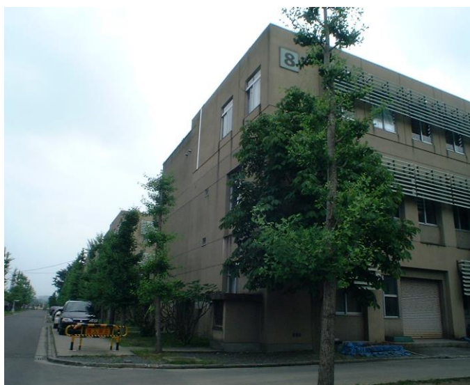
Appearance of Building
