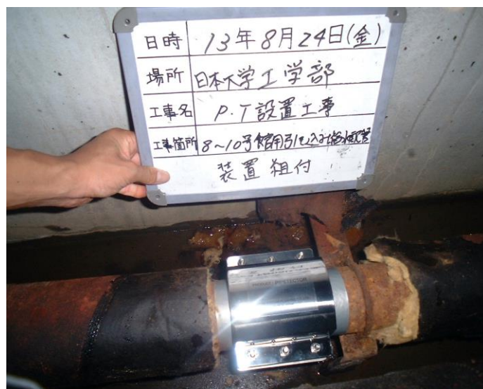
Installed on the water supply pipe
