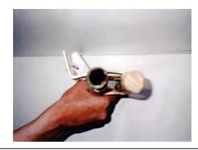
9 months after the installation The corrosion was reduced to magnetite and clogs of the cooling water pipe disappeared. So, the whole production line did not have to be stopped.
