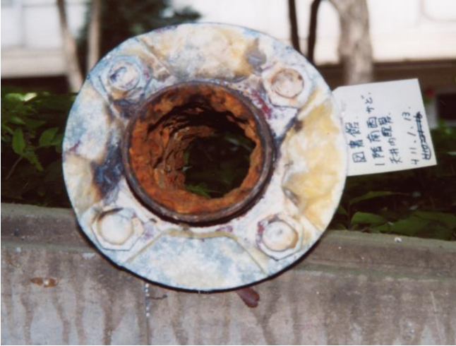
(Pipe cut on January 13 in 1999)
