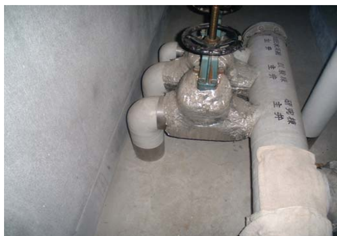
On outlet pipe of elevated water tank for the research building
