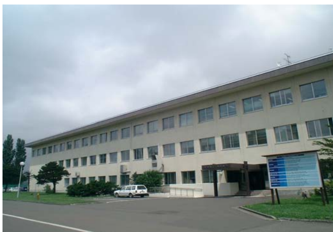
Appearance of Building
