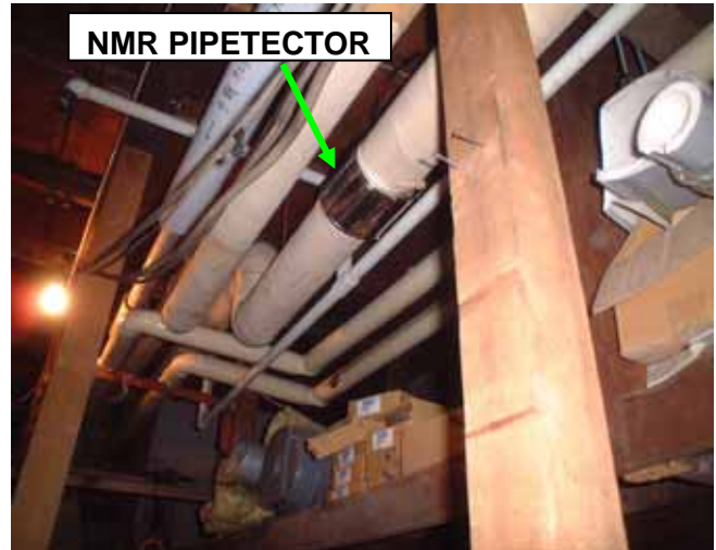
Outlet pipe of the boiler
