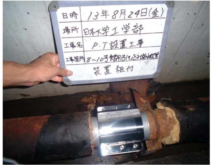
Installed on the water supply pipe
