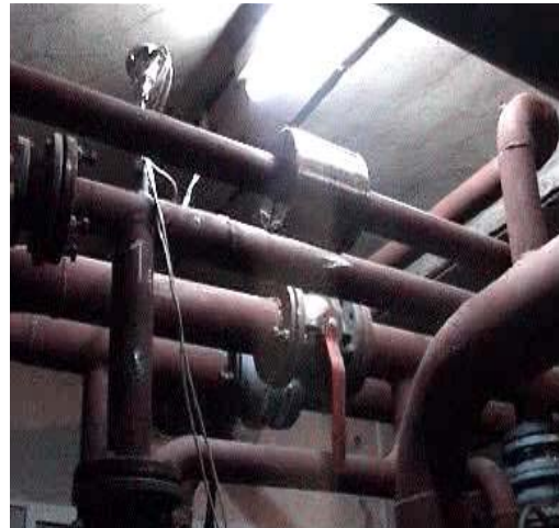
On outlet of hot water supply pipe PT- 50DS
